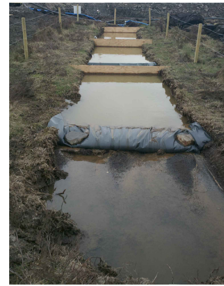
Completed Settling Pond System
